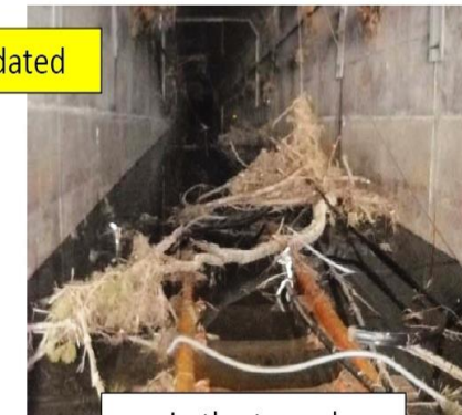
In the tunnel
